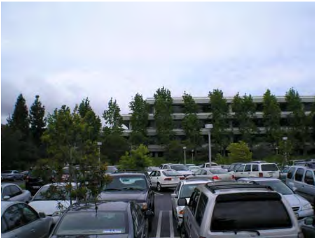
Southern portion of AT&T Building
