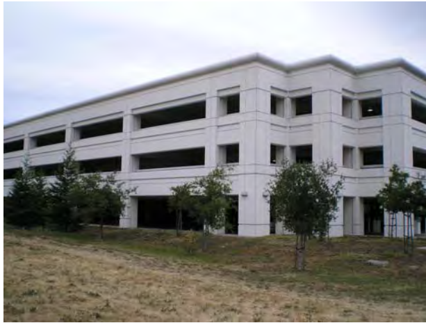
Northeast corner of project site - looking northwest
