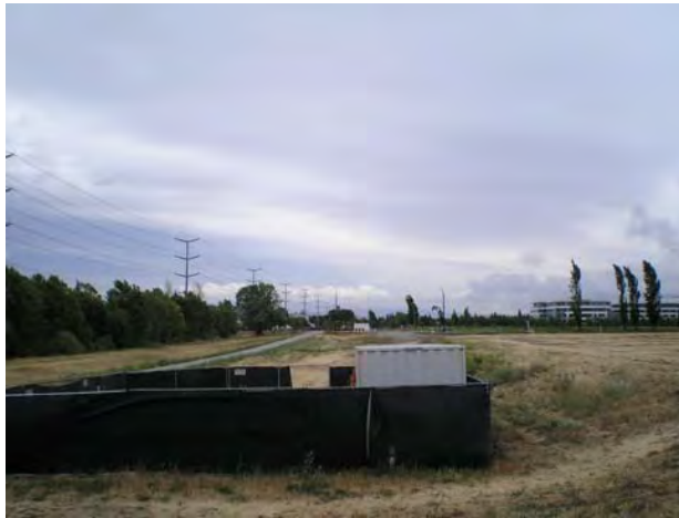
Northeast corner of project site - looking south
