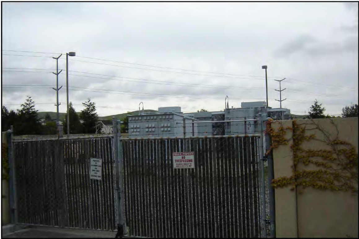
Photograph 1: Looking south at the utility corridor located just east of the southeast corner of the project site
