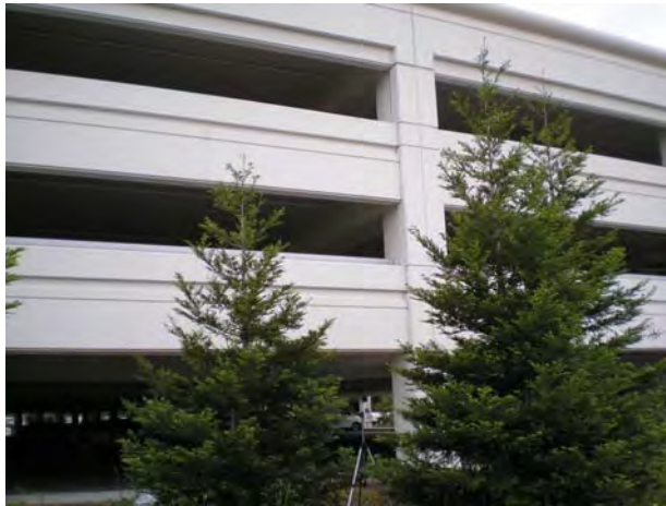
Noise Measurement Site B - looking north
